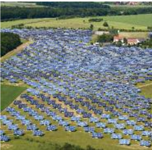
image THIS GERMAN SOLAR FARM IS THE LARGEST OF ITS KIND IN THE WORLD, WITH 1500 PHOTOVOLTAIC PANELS.
