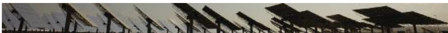
image THE PS10 CONCENTRATING SOLAR TOWER PLANT USES 624 LARGE MOVABLE MIRRORS CALLED HELIOSTATS. THE MIRRORS CONCENTRATE THE SUN'S RAYS TO THE TOP OF A 115 METER (377 FOOT)-HIGH TOWER WHERE A SOLAR RECEIVER AND A STEAM TURBINE ARE LOCATED. THE TURBINE DRIVES A GENERATOR, PRODUCING ELECTRICITY. SEVILLA, SPAIN.
