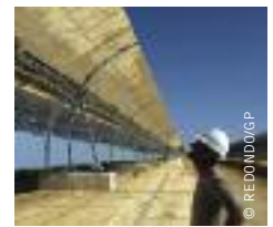
image THE PS10 SOLAR TOWER PLANT AT SAN LUCAR LA MAYOR, OUTSIDE SEVILLE, SPAIN, APRIL 29, 2008.
