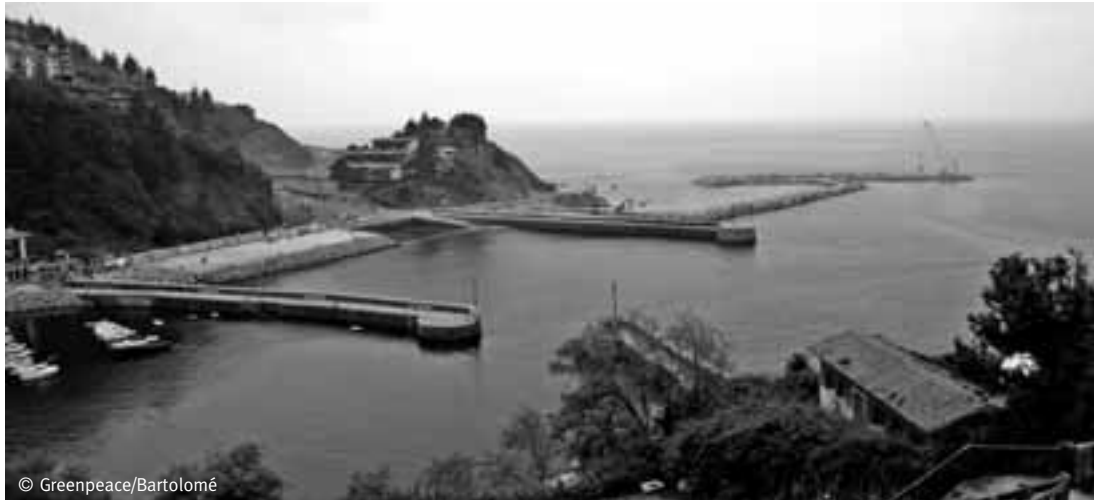
Expansion works in Port of Mutriku, Gipuzkoa.
