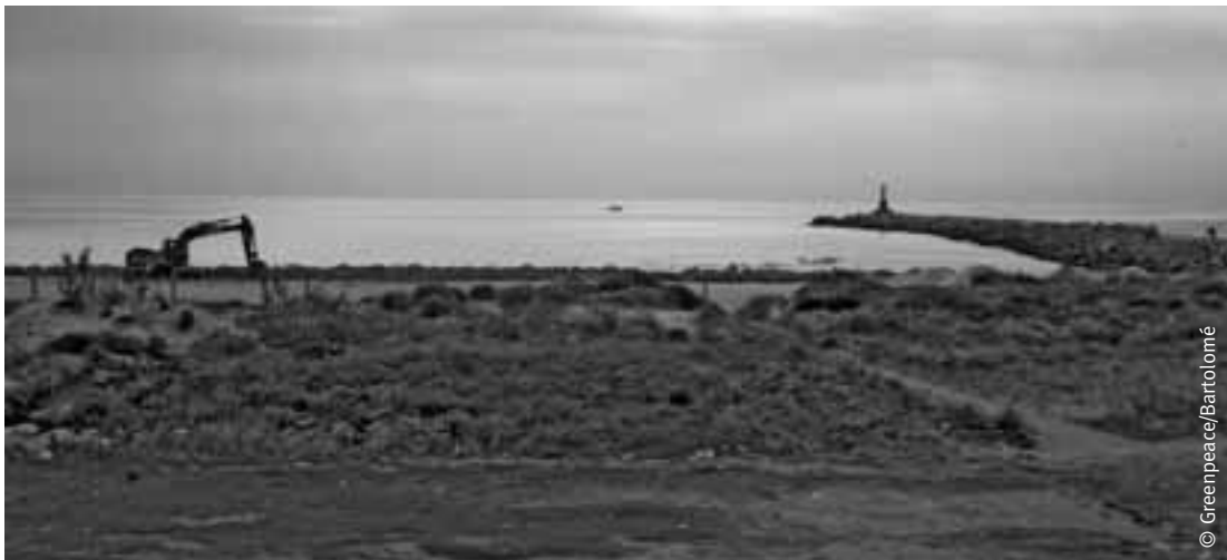
Machinery working on the sand in Escollera Beach, Cullera (Valencia).
