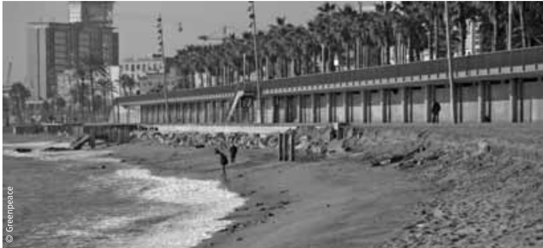
Erosion in La Barceloneta Beach, Barcelona.
