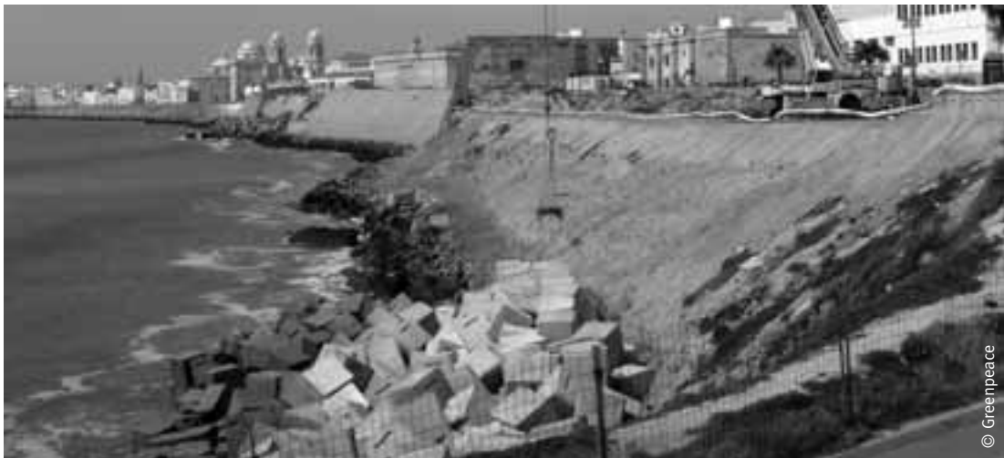
Concrete blocks to fight erosion in Cádiz.
