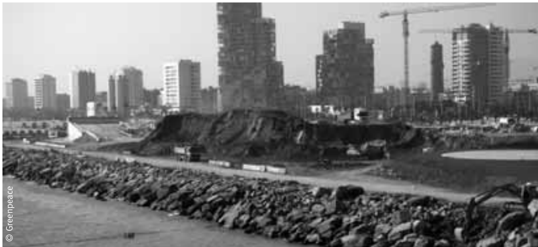
Construction of the Barcelona zoo, invading the sea.
