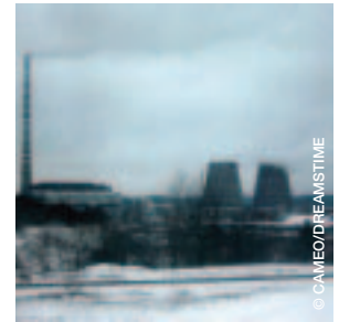
image A power generation plant near Vilnius, Lithuania on a cold winter's day.
