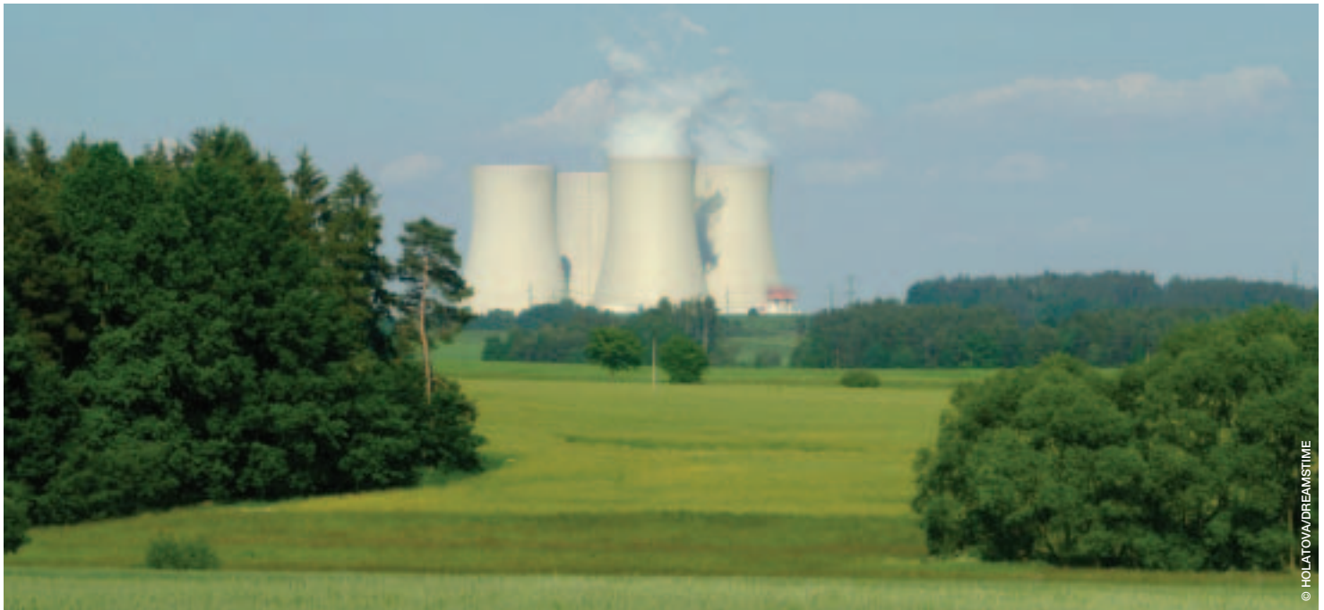
image Cooling towers of the nuclear power station Temelin in the Czech Republic.
