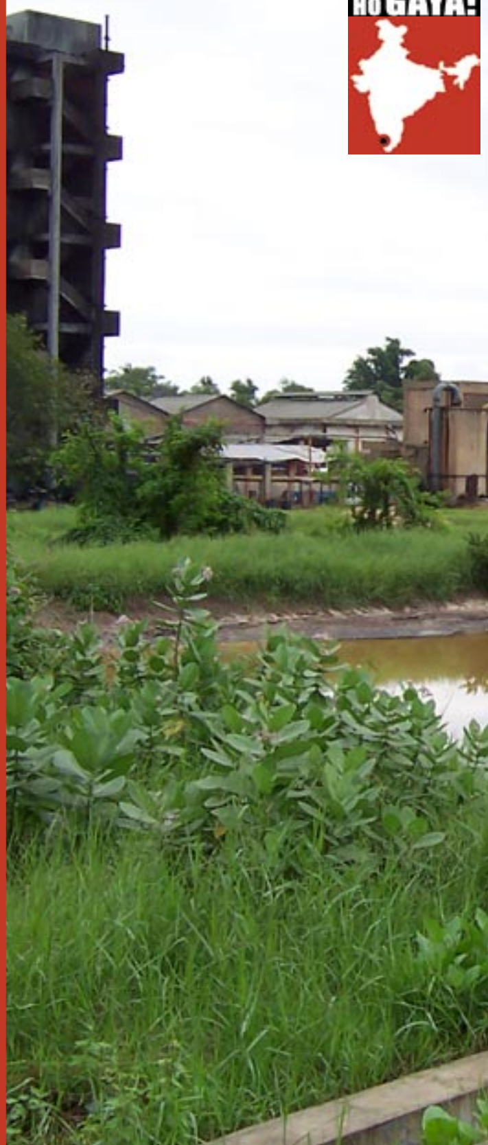
The soot-blackened building of Hindustan Insecticide Limited's endosulfan plant in Eloor. Picture by Nityanand Jayaraman.
