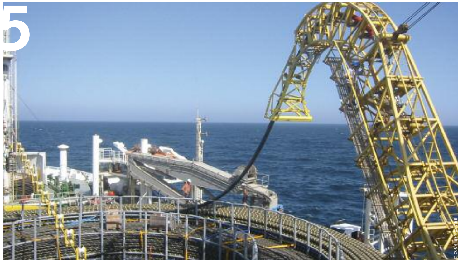
image LAYING SUBMARINE CABLE
