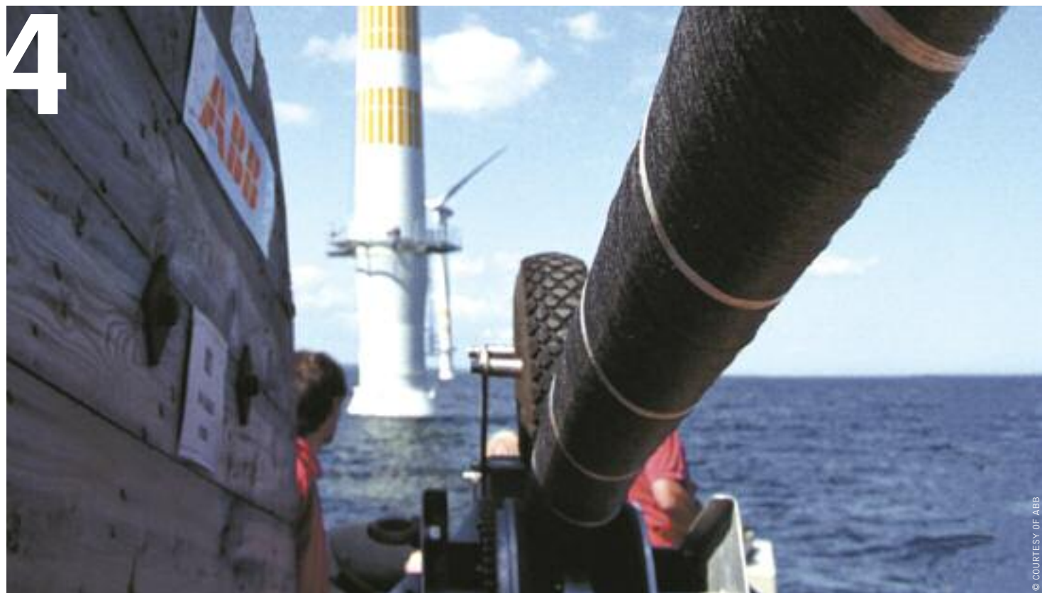
image SUBMARINE CABLE BEING CONNECTED TO A WINDFARM.
