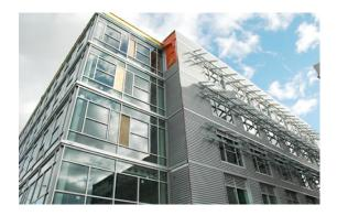
Office building in Seattle, Washington, designed by Weber & Thomson, requires no air-conditioning. The building has green-tinted glass shades (or sunglasses) that shield windows from heat, while still allowing light into the building. Heat-reflective coating on the windows also reduce temperatures. The 40,000 square foot structure has a central courtyard, which allows cross breezes to enter all parts of the building, and allows more natural light into the building. <sup>178</sup>
