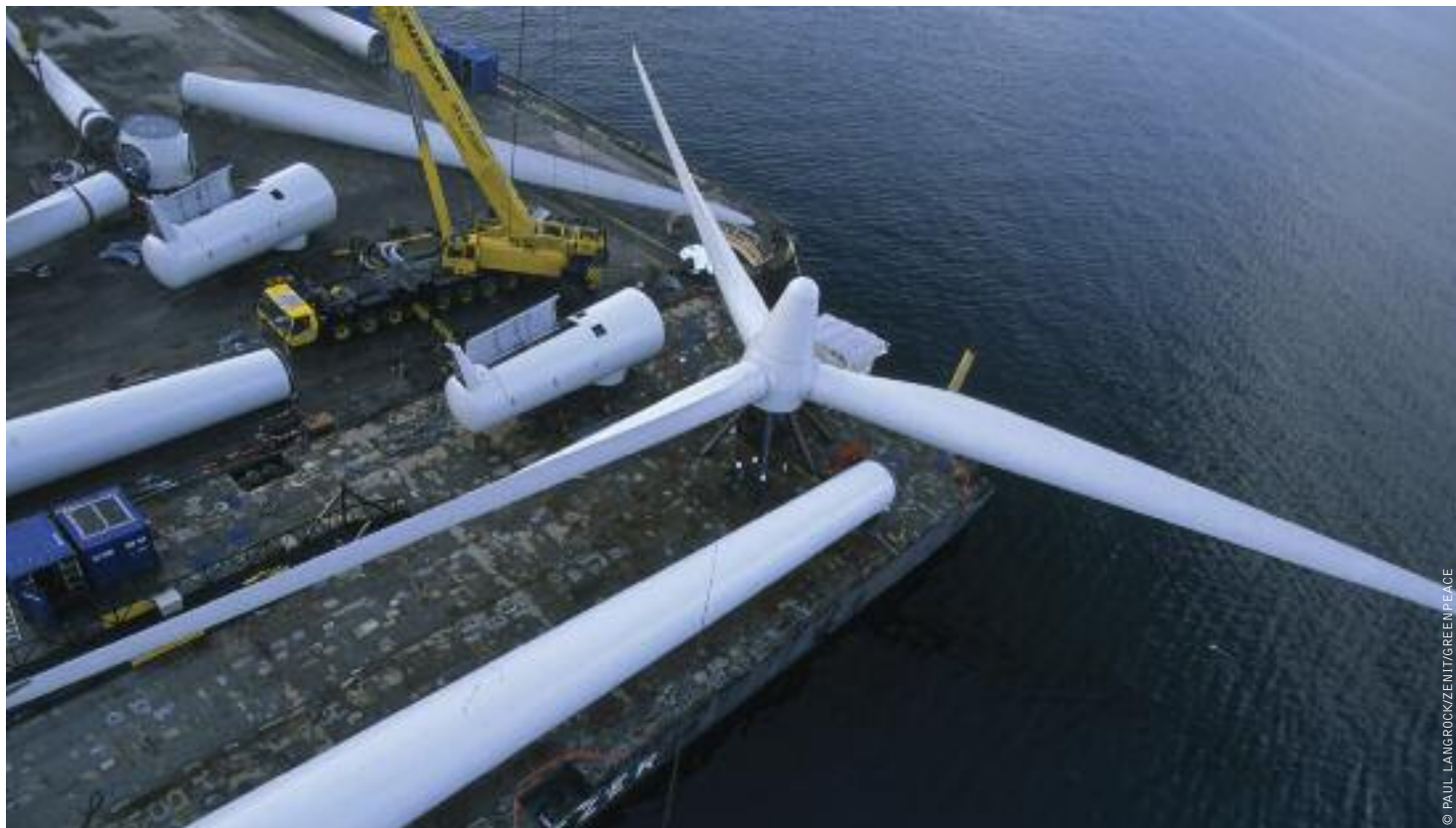
image CONSTRUCTION OF THE OFFSHORE WINDFARM AT MIDDELGRUNDEN NEAR COPENHAGEN, DENMARK.
