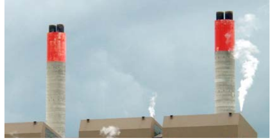
Huntly power station. Coal burning emits atmospheric pollutants and coal mines destroy landscapes and poison waterways.
