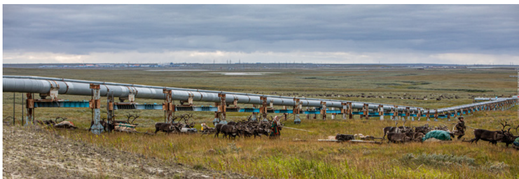
Russian pipeline crossing Nenets' traditional lands.
