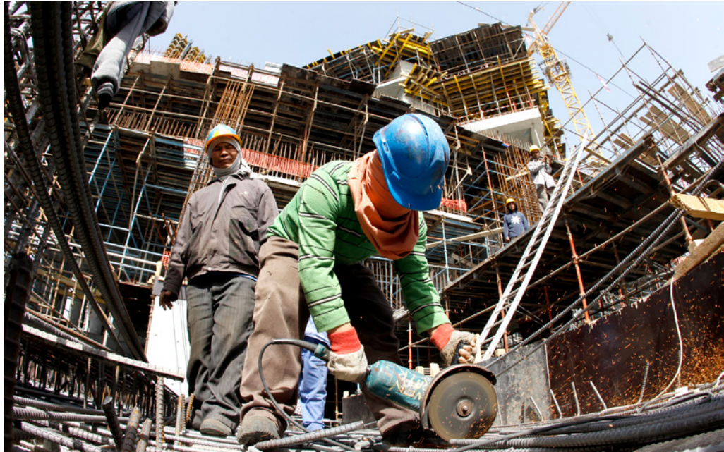
A migrant worker cuts through a metal rod at a construction site.
