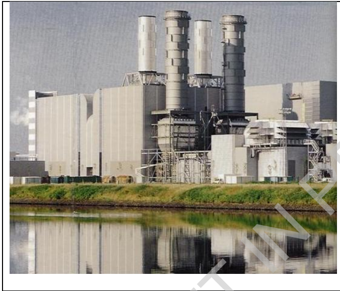
Figure 2.16: Recently built gas turbine combined cycle power plant in Belgium
