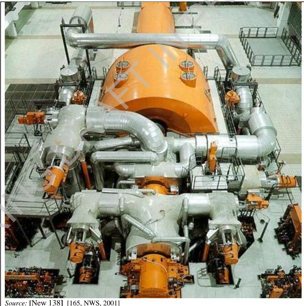
Figure 2.17: Steam turbine of a coal-fired power plant
