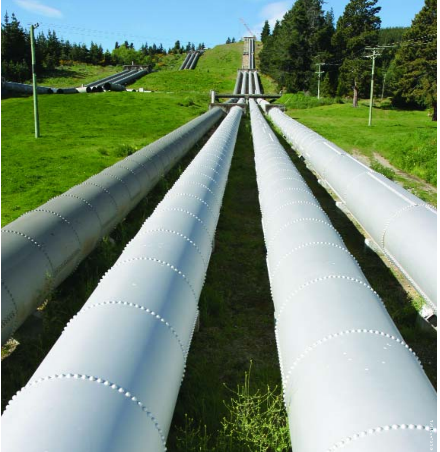
image HOT-RIVETED STEEL PENSTOCKS AT AN OLD HYDRO-ELECTRIC POWER STATION, LAKE COLERIDGE, CANTERBURY, NEW ZEALAND.
