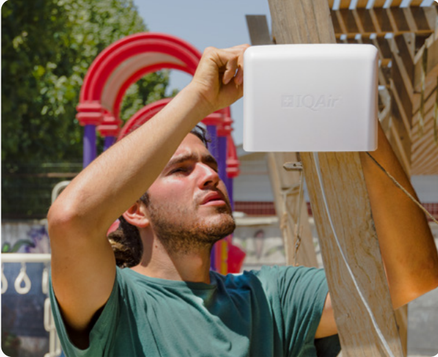
Community member installing an air quality sensor near a playground
