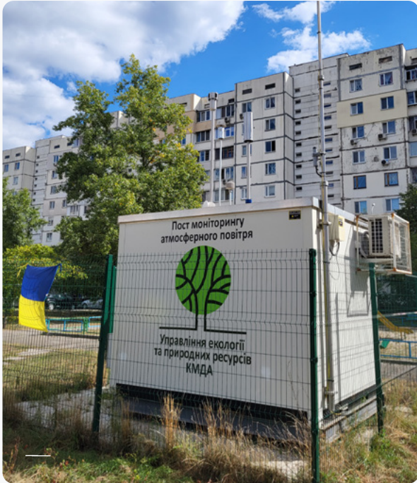
Official Kyiv city air quality monitoring station.
