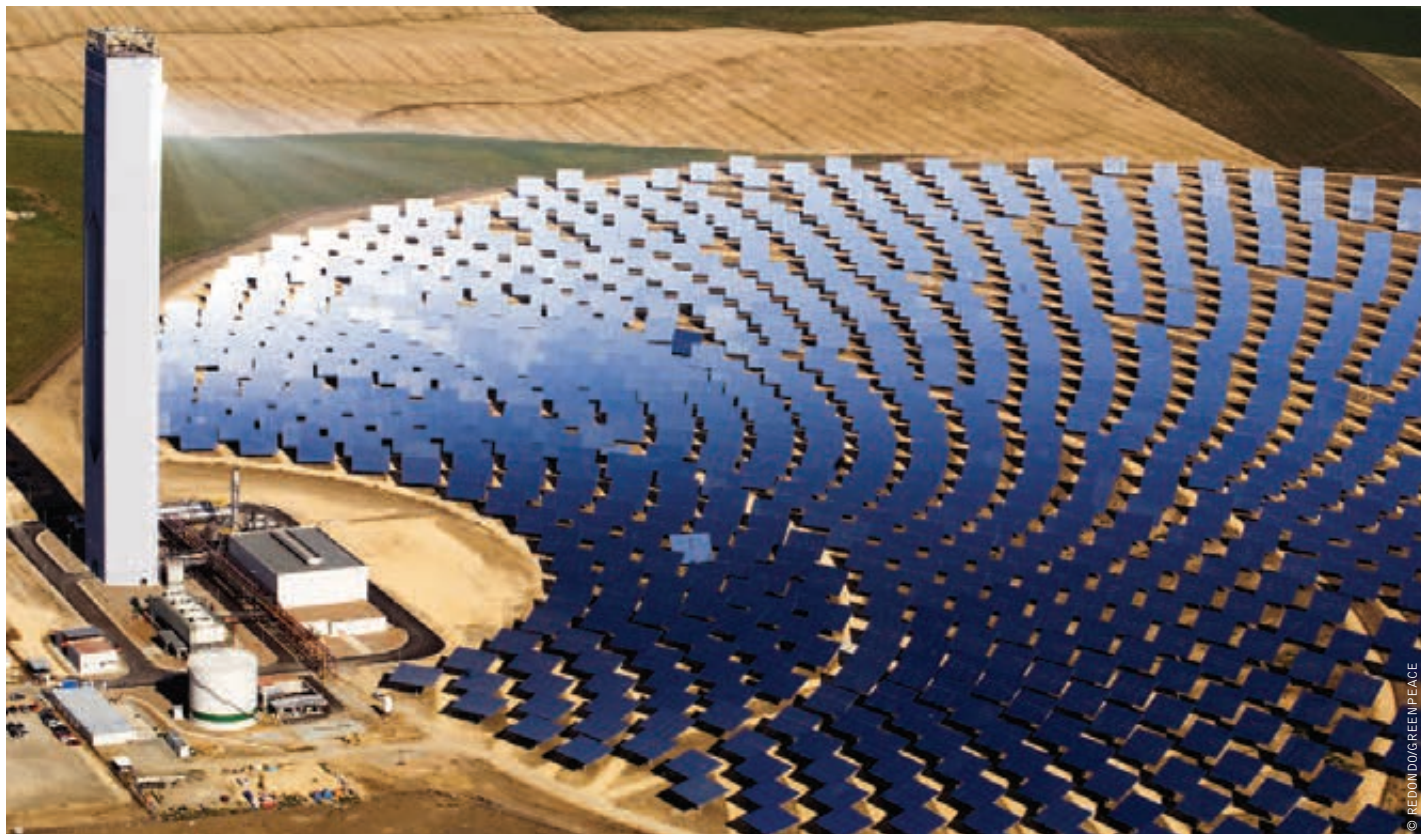
image AERIAL PHOTO OF THE PS10 CONCENTRATING SOLAR THERMAL POWER PLANT. THE 11 MEGAWATT SOLAR POWER TOWER PRODUCES ELECTRICITY WITH 624 LARGE MOVABLE MIRRORS CALLED HELIOSTATS. THE SOLAR RADIATION, MIRROR DESIGN PLANT IS CAPABLE OF PRODUCING 23 GWH OF ELECTRICITY WHICH IS ENOUGH TO SUPPLY POWER TO A POPULATION OF 10,000.
