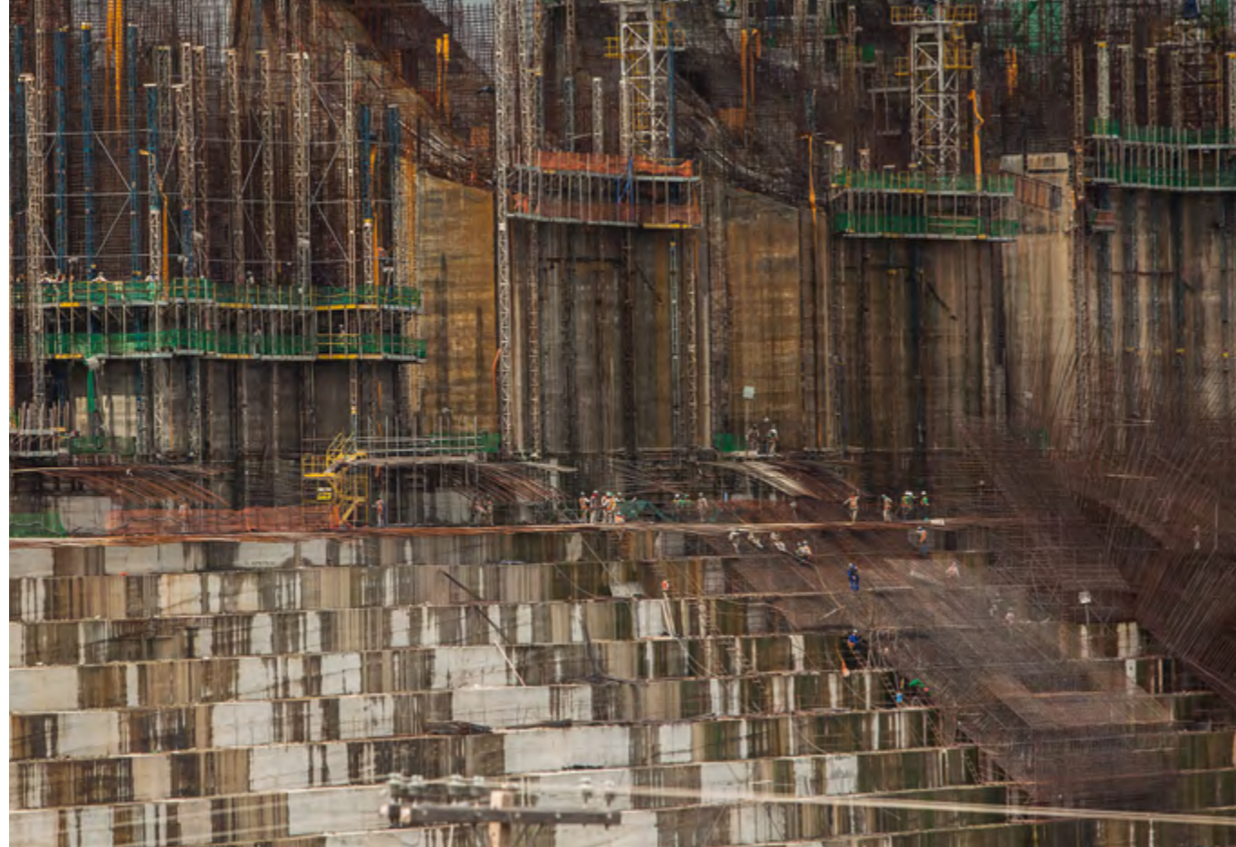
Construction of the Belo Monte hydropower complex, Pará State.. © Carol Quintanilha/Greenpeace
