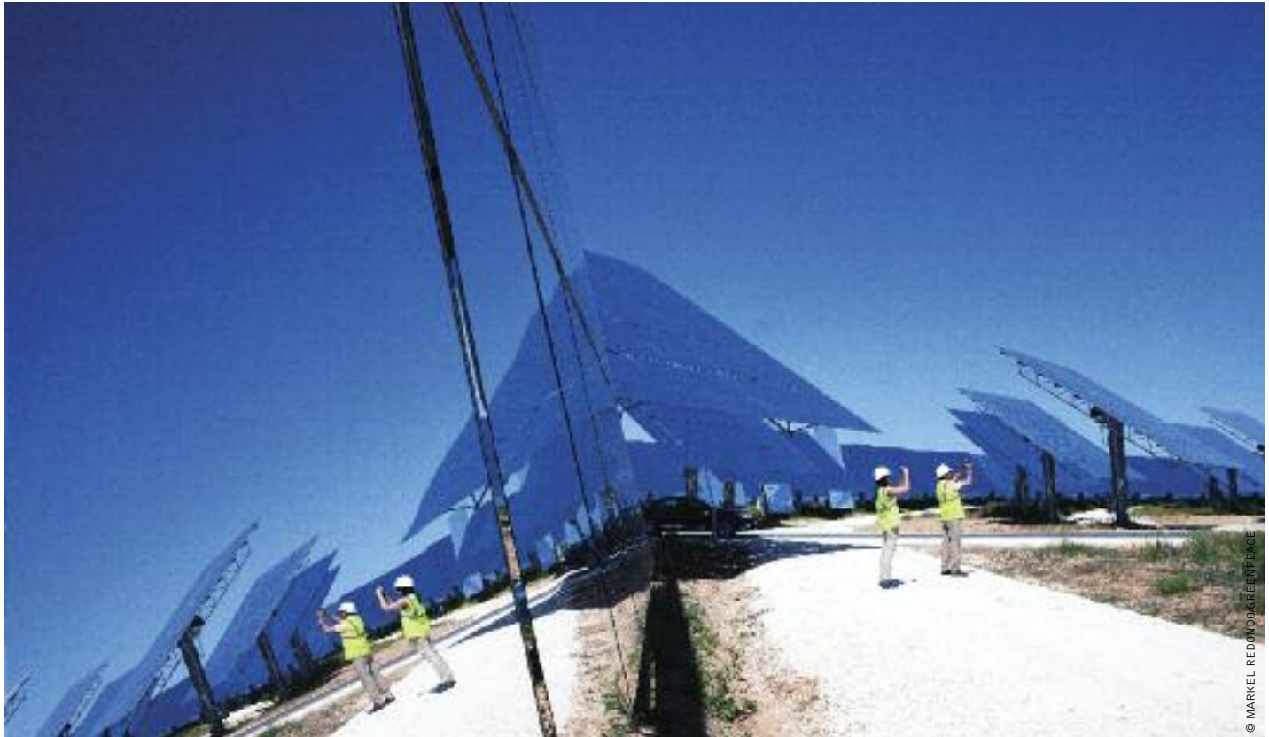
image GEMASOLAR, A 15 MWE SOLAR-ONLY POWER TOWER PLANT. IT'S 16-HOUR MOLTEN SALT STORAGE SYSTEM CAN DELIVER POWER AROUND THE CLOCK. IT RUNS THE EQUIVALENT OF 6,570 FULL HOURS OUT OF A 8,769 TOTAL. GEMASOLAR IS OWNED BY TORRESOL ENERGY AND HAS BEEN COMPLETED IN MAY 2011.
