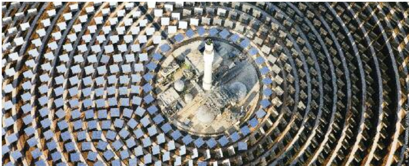
IMAGE GEMASOLAR, A 15 MW SOLAR POWER TOWER PLANT, SPAIN.
