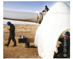
image MAINTENANCE WORKERS FIX THE BLADES OF A WINDMILL AT GUAZHOU WIND FARM NEAR YUMEN IN GANSU PROVINCE, CHINA.
