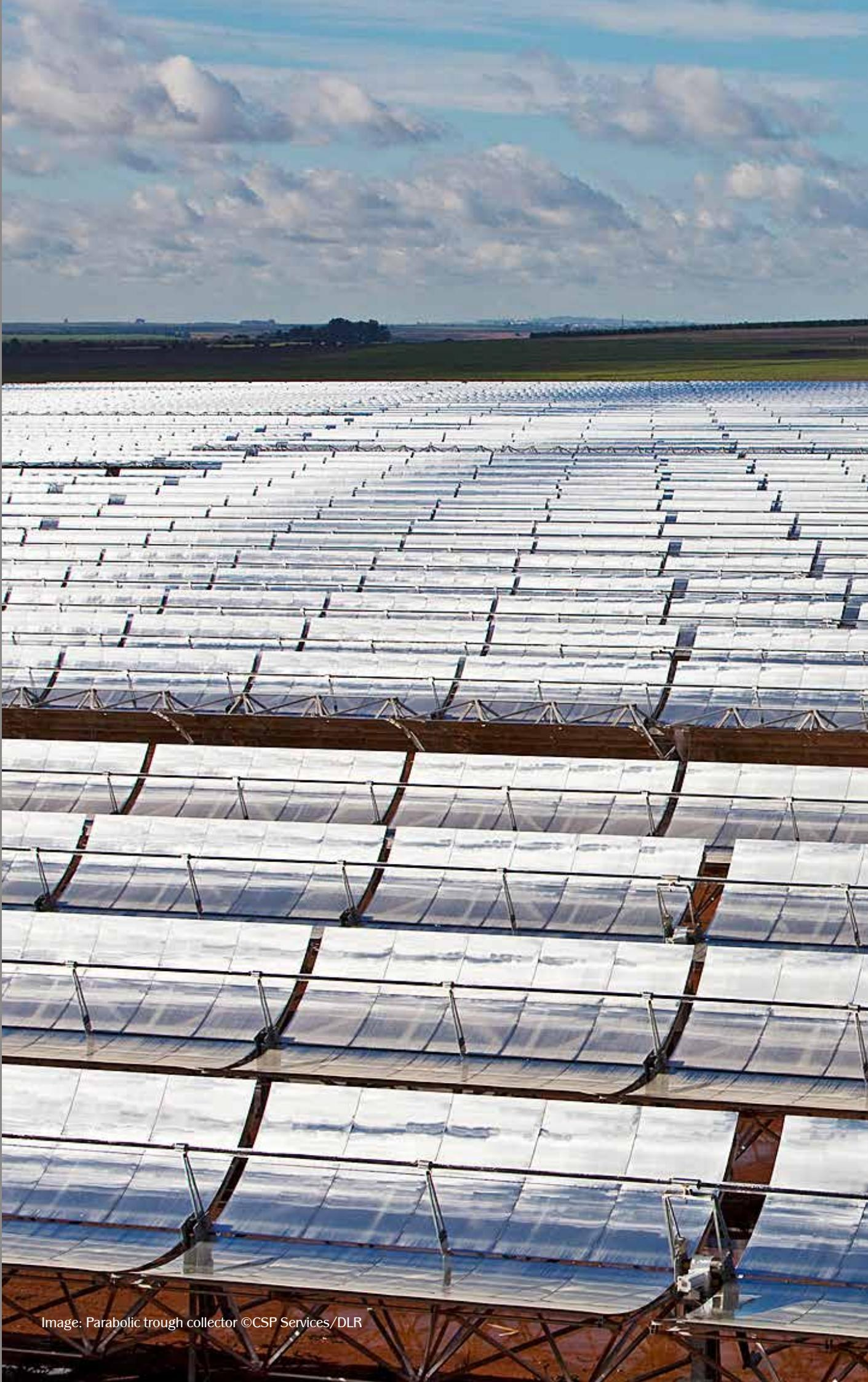
Image: Parabolic trough collector ©CSP Services/DLR
