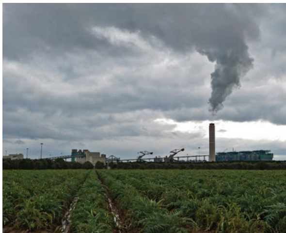
BRINDISI POWER PLANT. © Ida Santoro
