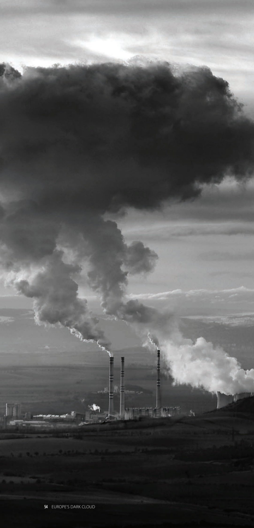
POČERADY POWER PLANT, CZECH REPUBLIC. © zahorec
