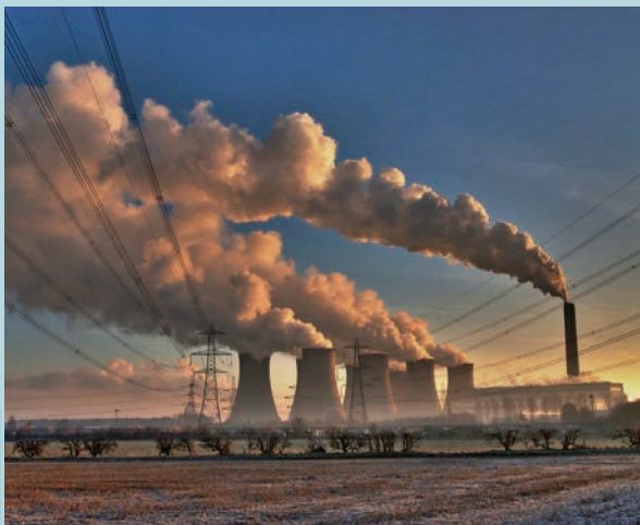
EGGBOROUGH POWER PLANT. © John Mabbitt
