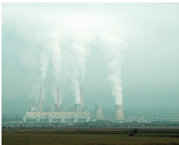
AGRIOS DIMITRIOS POWER PLANT. © Ioannis Tokaris
