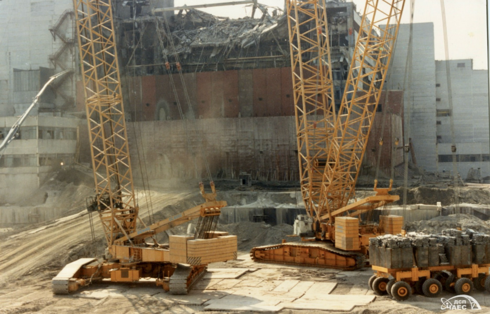
Demag cranes during construction of shelter in 1986 – Credit ChNPP
